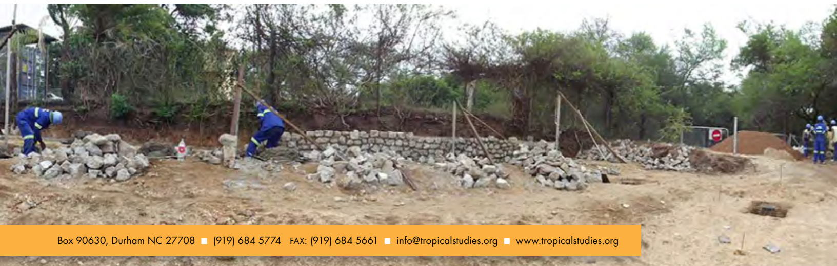
The initial walls were built using recycled concrete slabs rather than using new bricks. SANParks (South African National Parks) engineers chopped up the old helicopter landing pad/parking lot on the site and produced chunks which were used for the project.
