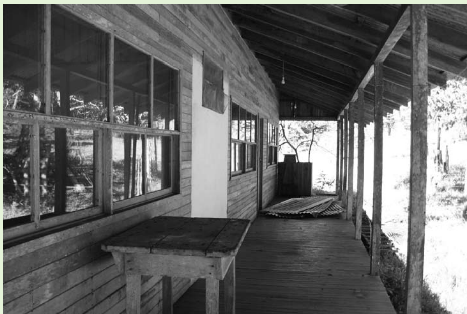
The corridor of the rustic Las Alturas field station, soon to be repaired and expanded. Photo Zak Zahawi.
