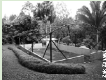
The Cactus Greenhouse under construction.
