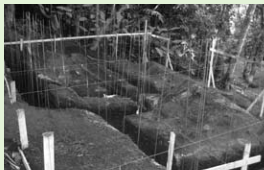
The excavation for one of the new researcher cabins under construction. Photo Zak Zahawi.
