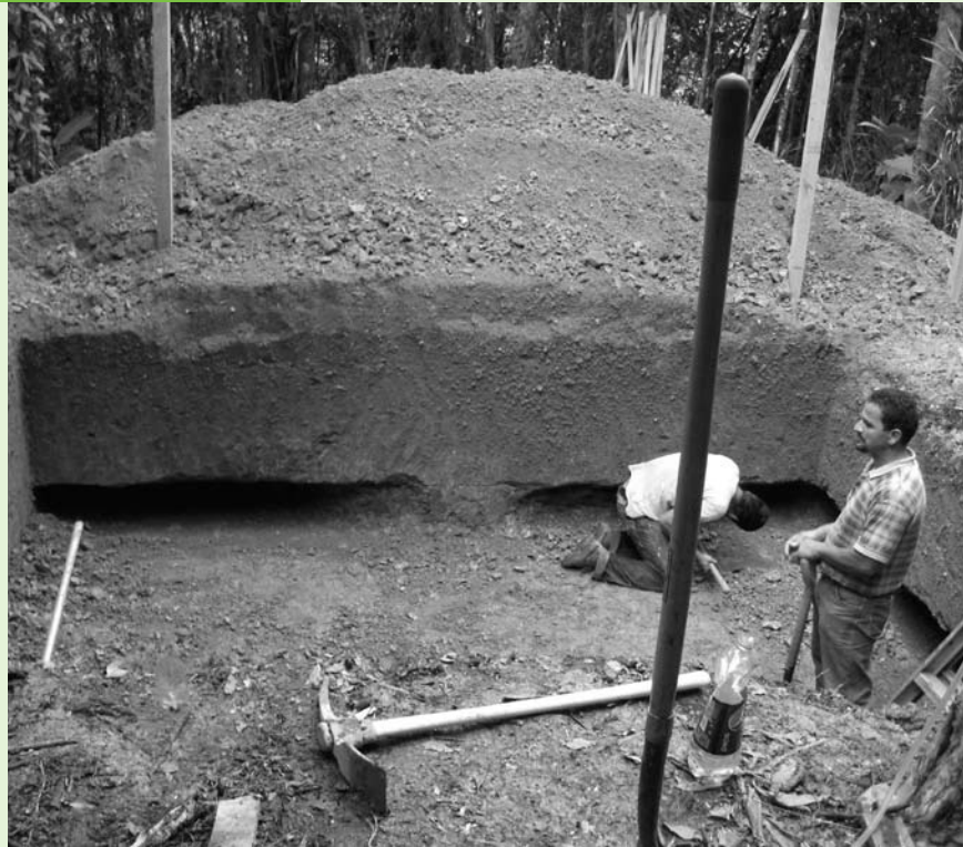
The freshly dug pit from which the Las Cruces canopy tower will soon emerge! Photo Zak Zahawi.
