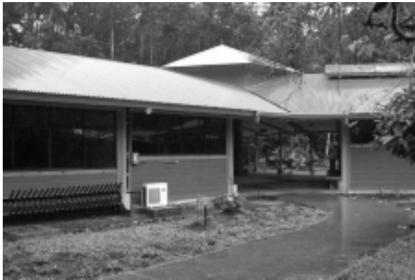
A new education building was constructed at La Selva to provide dedicated space for courses.
